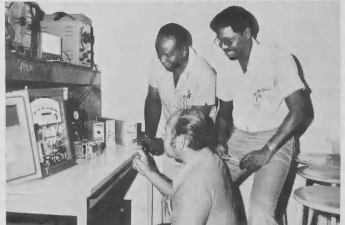
at far right among an array of pneumatic and electronic control instruments. The CMA is the latest development in Direct Digital Computer control.
